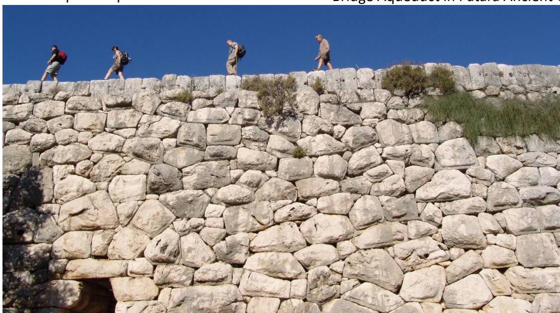
Walking on top of the Siphon Aqueduct
